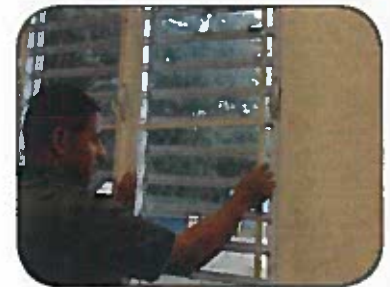
Install or repair window & door screens.
